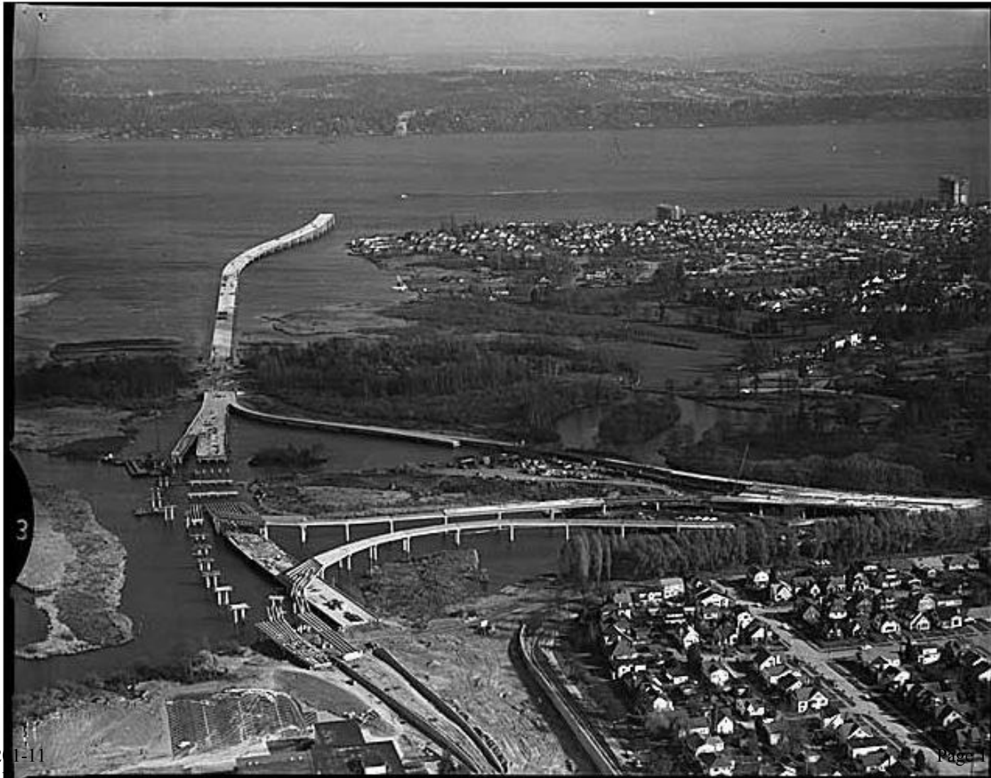
Aerial of Evergreen Point Bridge under construction from west, Seattle, 1963
