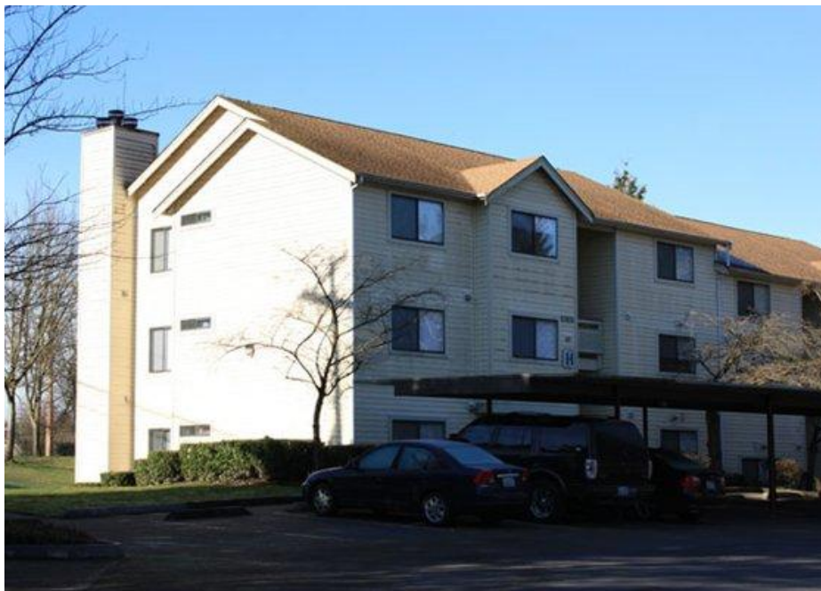
Figure 2. A student residence building at the complex
