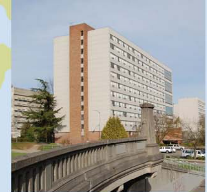
Existing Terry Hall from University Bridge
