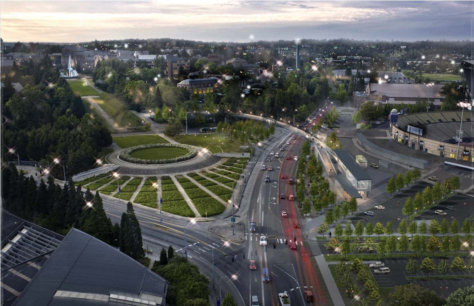
STATION AERIAL VIEW
